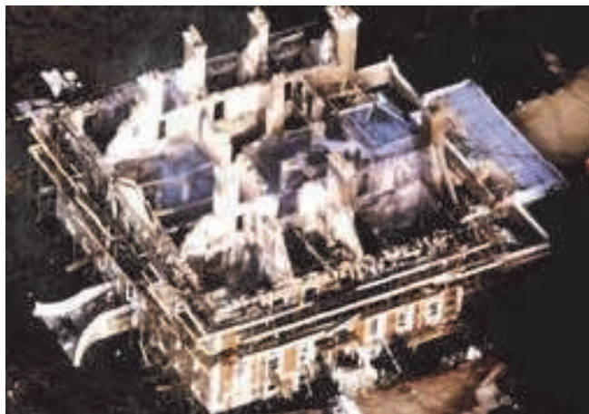
Fires in Historic Buildings frequently cause complete destruction!
