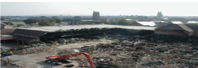
The consequences of a serious fire in an un-sprinklered supermarket. The building was rebuilt with sprinkler protection
