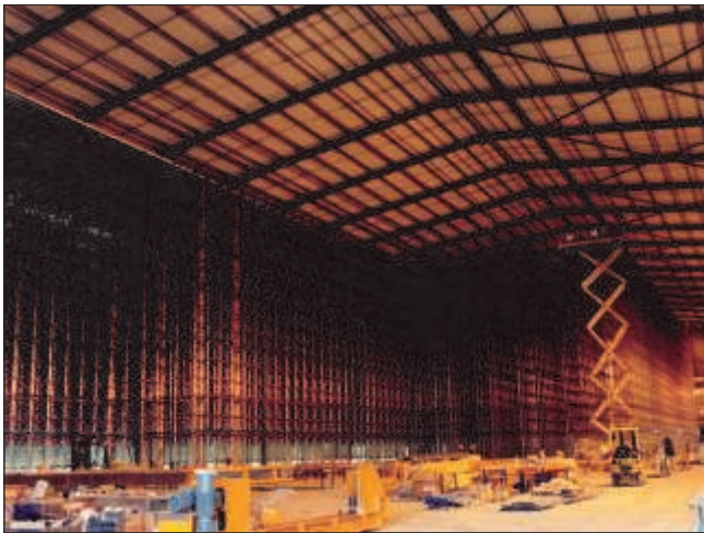
Installation of High-Bay racking.
