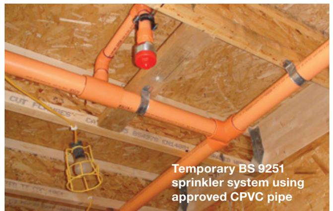
Temporary BS 9251 sprinkler system using approved CPVC pipe
