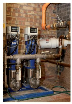
The four internal service mains in the block provided the water for the sprinkler system. Twin electric pumps supplement the service main's supply although, during installation, the mains pressure was tested and the 1.5bar reading at the top floor was in any case judged sufficient for the system.
