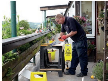
Preparation and fitting Pendoc boxing
