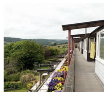
Felt covered timber walkway on top floor
