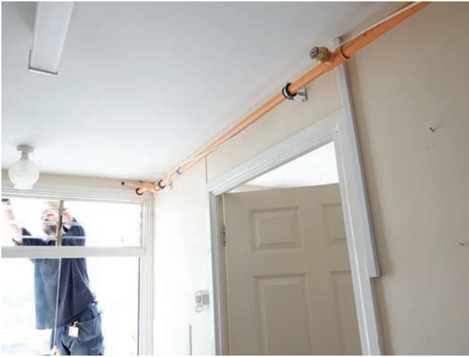
Installation of CPVC pipework
