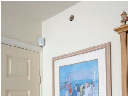
Sprinkler installation prior to fitting cover plate
