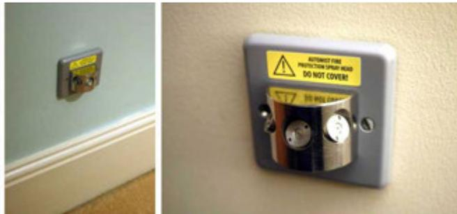
Figure 6: Electronically Controlled Nozzle Example
