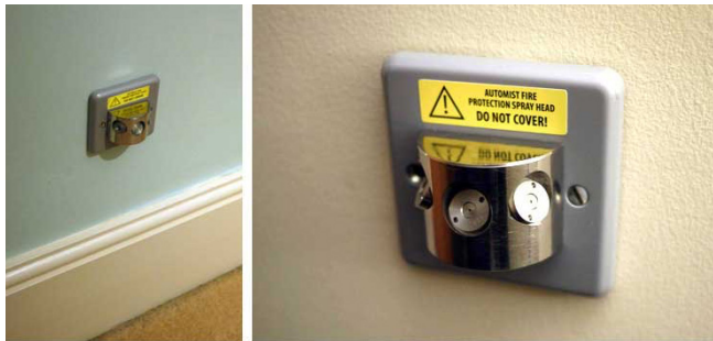
Figure 6: Electronically Controlled Nozzle Example
