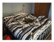
gone through to the kitchen where he had an epileptic fit. The bed subsequently caught fire due to smoking materials. Nearby residents were alerted to the fire by the alarms. (both Smoke and Sprinklers) A single sprinkler head operated and fully extinguished the fire before the Fire Brigade arrived. Fire Brigade personnel had to break into the flat to gain access, finding the occupant unconscious in the kitchen following his seizure.
