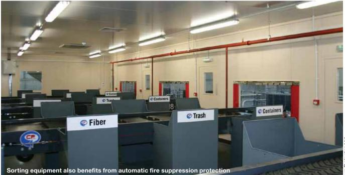
Deluge/waterspray systems should be designed to NFPA 15 or EN DD TS 14816.
