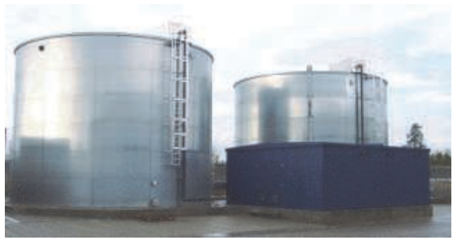
Typical sprinkler water supply with two tanks.
