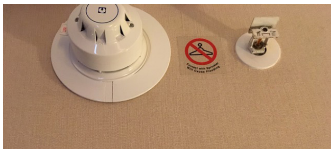
Retrofitted sprinkler system in an Grade II* hotel in Bristol. Note that warning sign - garment bags and sprinklers are not friends!
