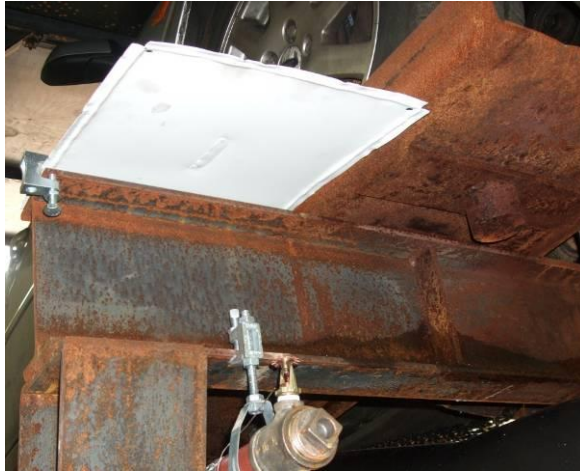
Figure 7 – Baffle plate installed above intermediate sprinkler head
