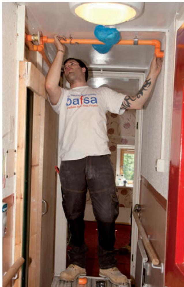
CPVC pipework and related components were the products of choice for the project. Some boxing-in would be necessary for system pipework although, wherever possible, it was hidden within the same concealment as domestic rising mains.
