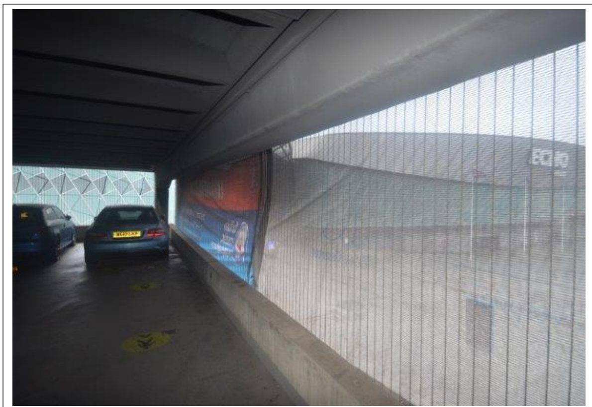
Figure 4.2: Internal view of grille and advertising on level 2
