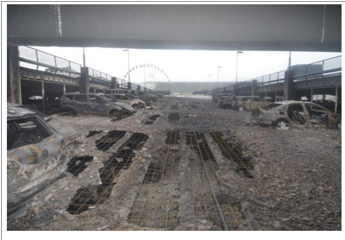
Figure 2.1.2: Photograph of ramp from level 6 to level 7
