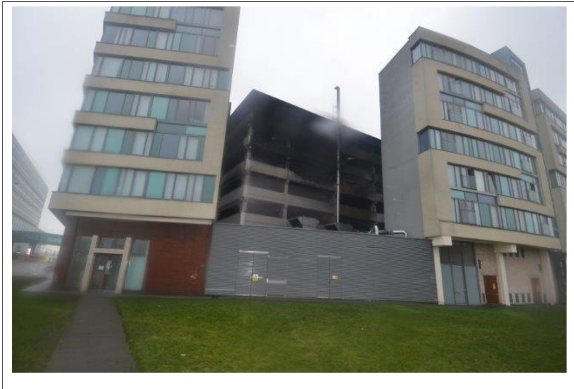
Figure 3.5.3: Firefighting Access on the eastern elevation, viewed from easterly direction
