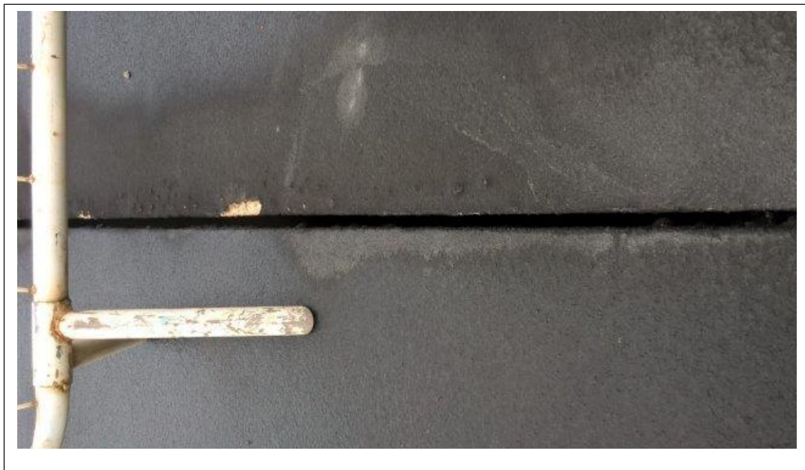
Figure 2.2.2: photo view of the drainage slot from above, Level 7 Roof
