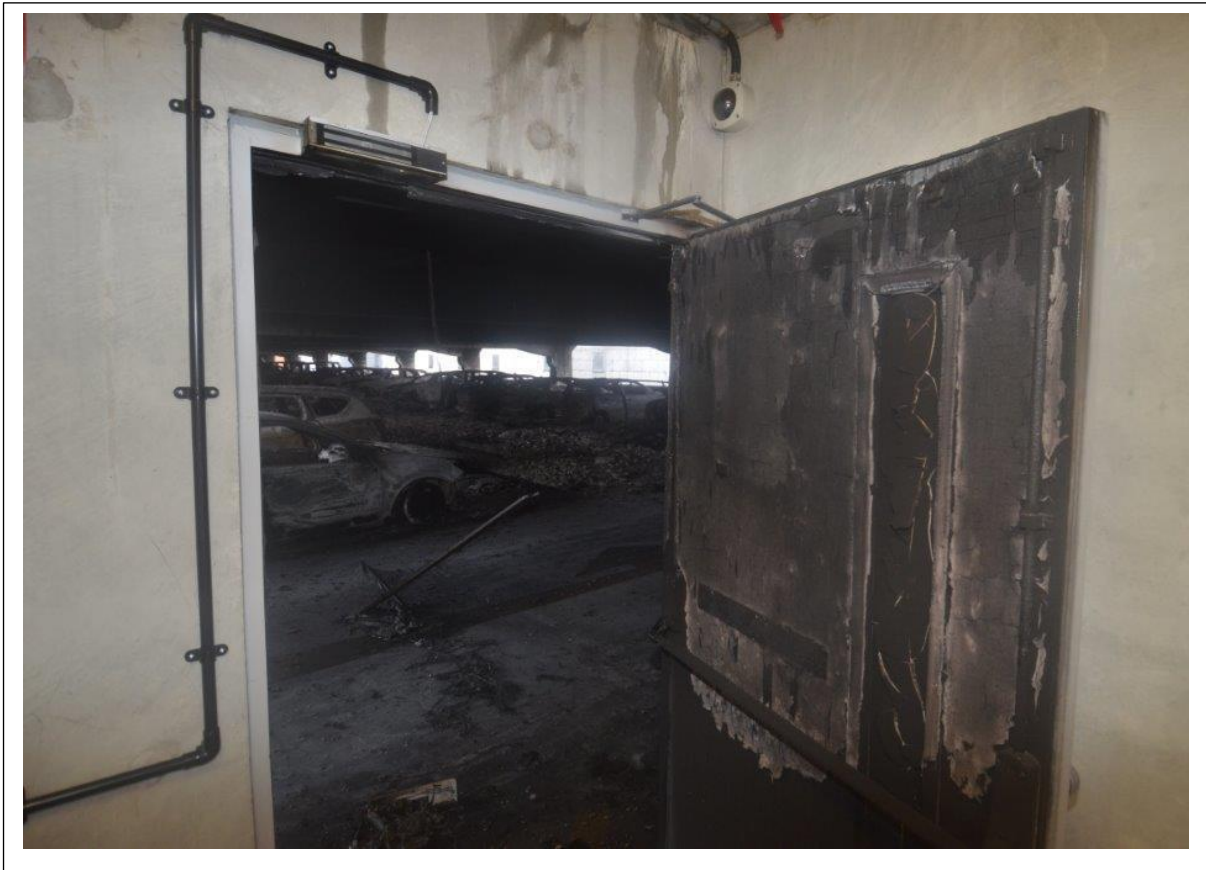
Figure 3.4.10 Stairwell 3 Level 2 exit from parking area
