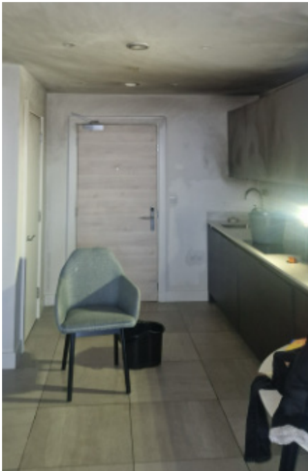
Image credit UK Sprinklers Ltd
