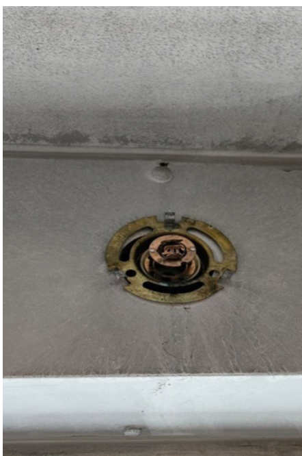
Sidewall sprinkler head Credit: ReCom fire protection ltd
