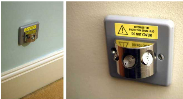
Figure 6: Electronically Controlled Nozzle Example
