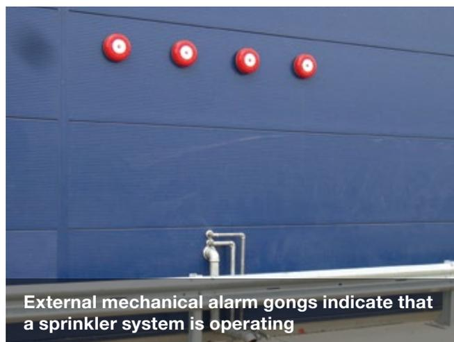
**External mechanical alarm gongs indicate that a sprinkler system is operating**
