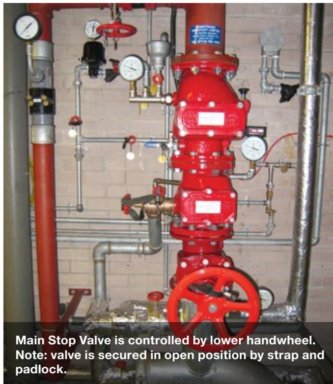
**Main Stop Valve is controlled by lower handwheel. Note: valve is secured in open position by strap and padlock.**
