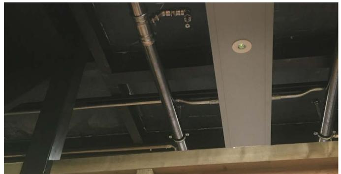
**Interior showing complex ceiling decor with mist nozzle. Pipework is visible to avoid fabric damage.**
