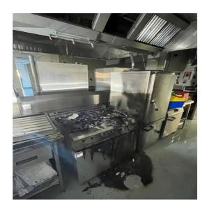
Due to the activation of a concealed sprinkler head fire damage at the school was minimal. Pic courtesy:
